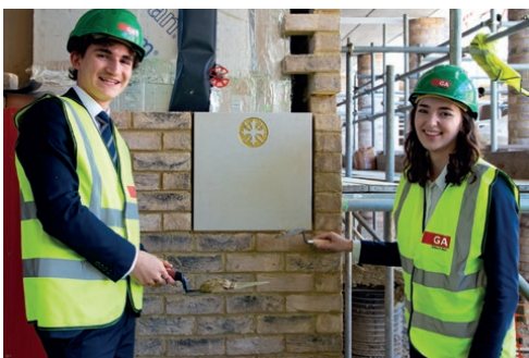
12 ▲ Head Prefects Sebastiano Zane and Millie Richardson with the foundation stone for the new Turberville Building, June 2018
