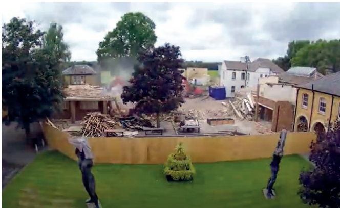
10 ▲ The demolition of the Jubilee Block in 2018
